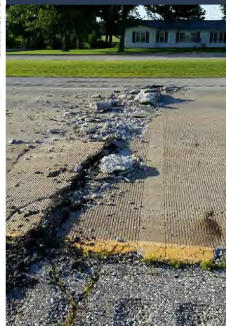
Road buckling caused by extreme heat June 2017 (photo: Illinois DOT via Flickr)
