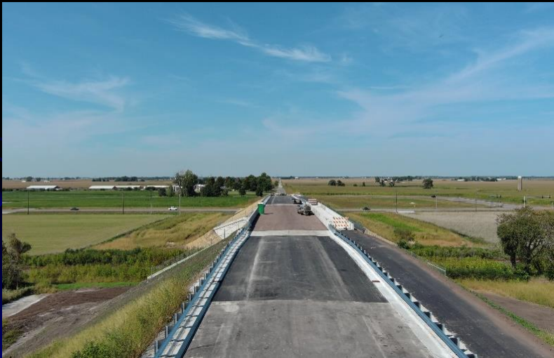
Crews work on final surface on the roadway and bike paths, installation of fencing, guardrail and landscaping on the Dauberman Road Extension project
