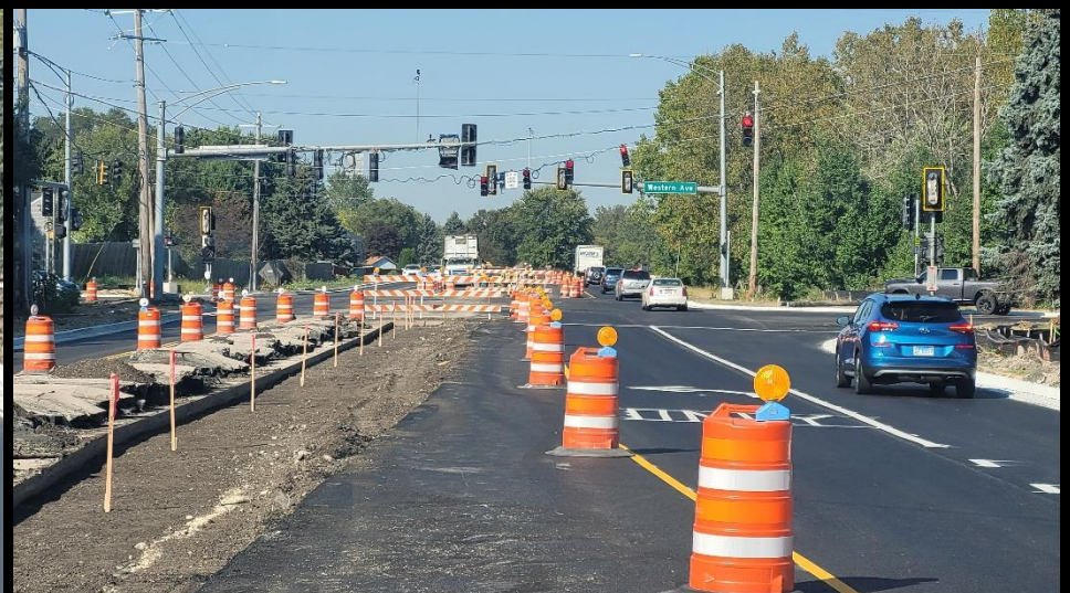
Crews work on base preparation, asphalt paving and new curb and gutter on the Fabyan Parkway at Western Ave Intersection Improvement
