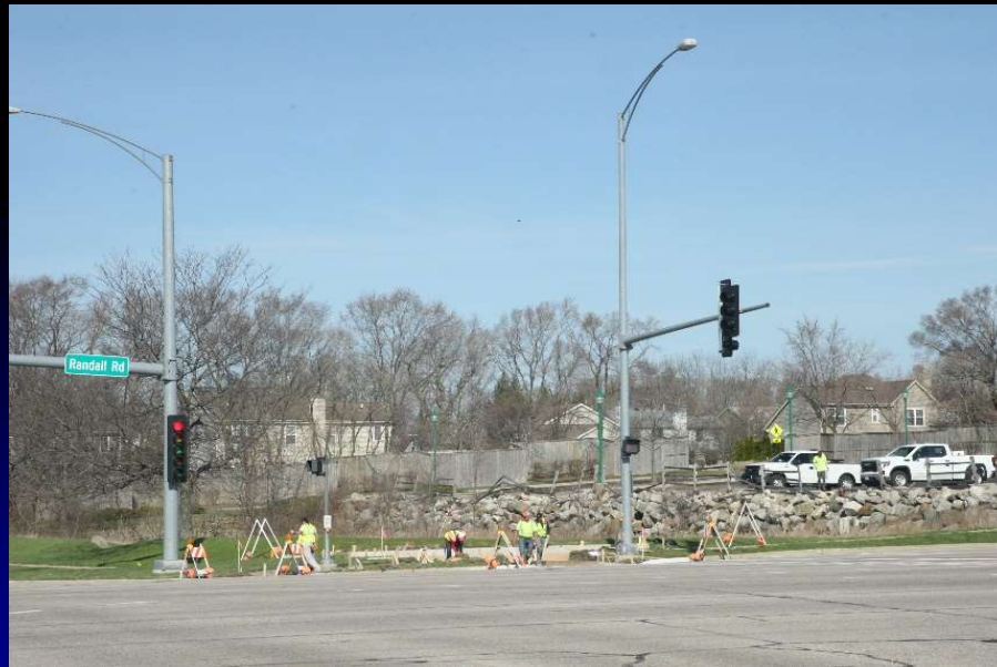
Crews employ proper traffic control as they remove and replace ADA ramps along Bowes Road as part of the 2023 ADA Improvement project
