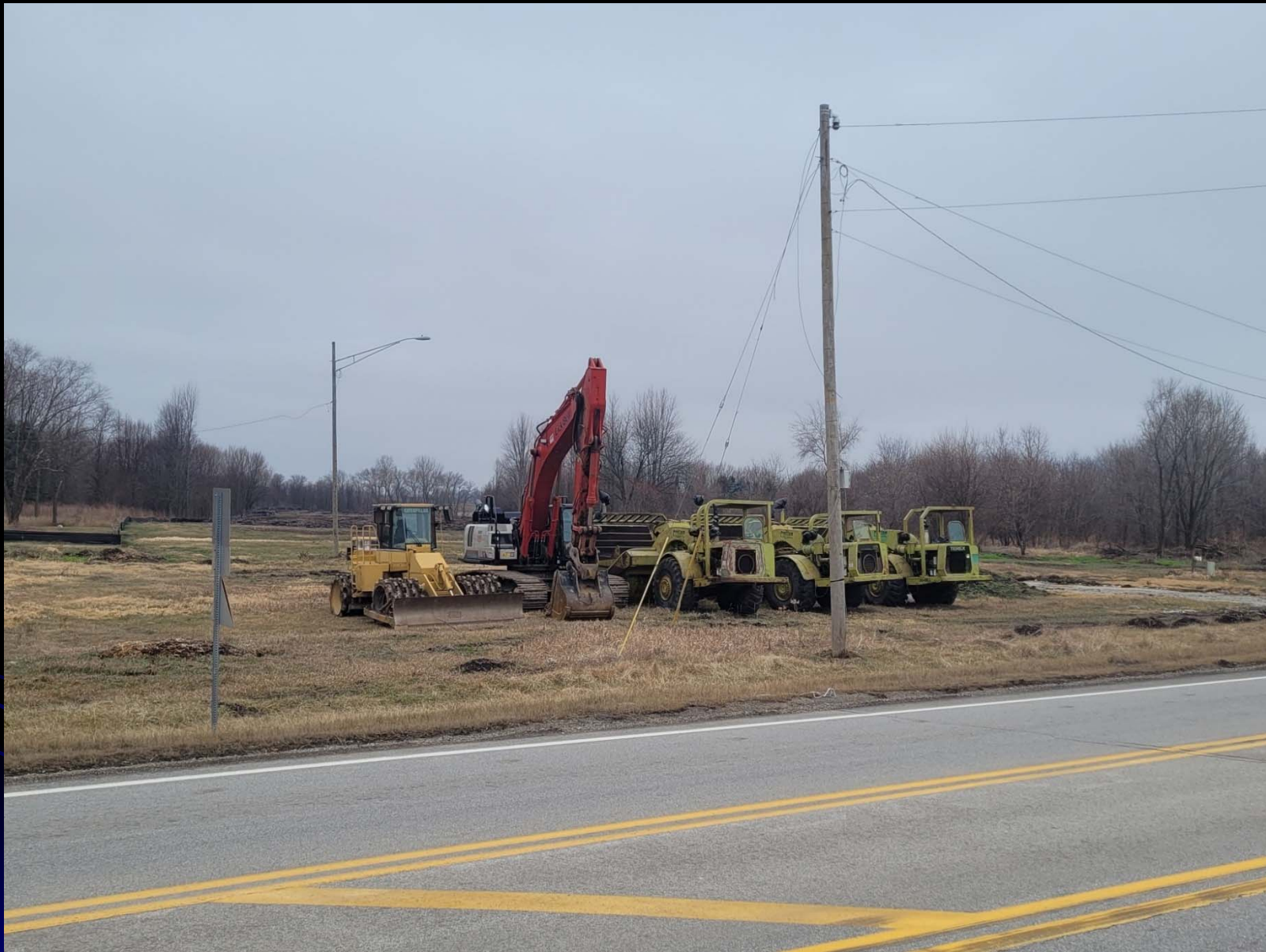
Earth moving equipment is ready in preparation for a box culvert installation on the Bliss/Main/Fabyan Intersection Improvement project
