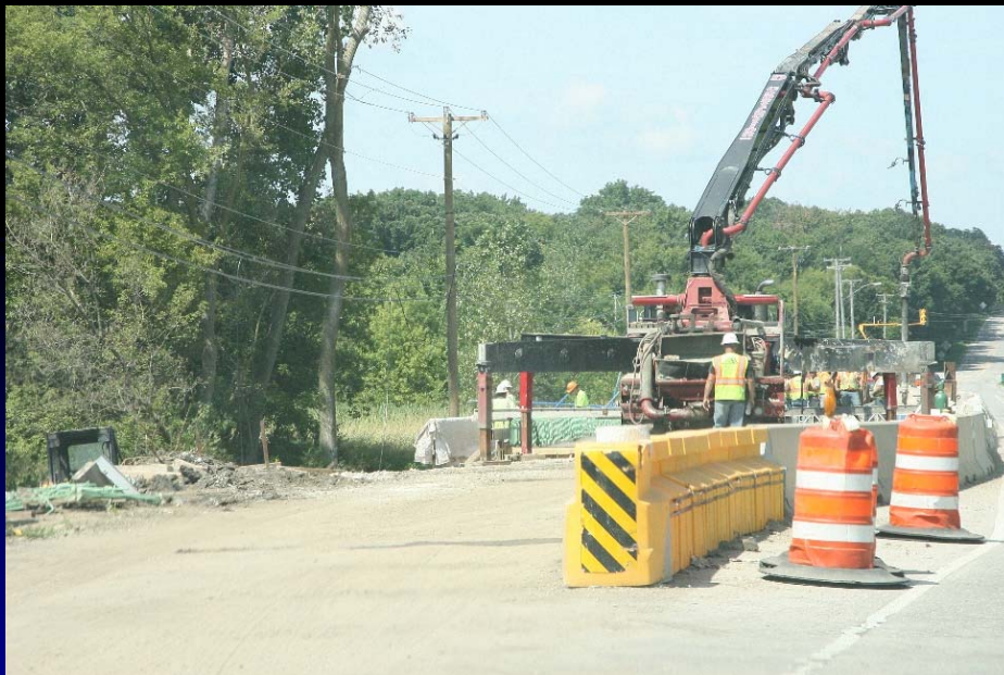
Crews place the rebar reinforcement mat and then complete the concrete pour for the new bridge deck on the Silver Glen over Otter Creek bridge replacement project
