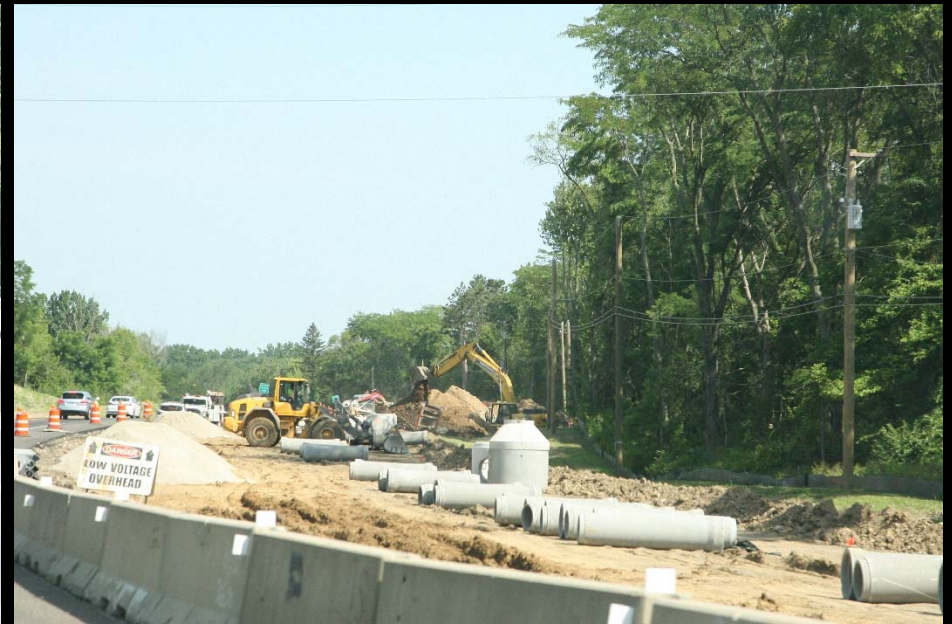
Crews installing new storm sewer along IL Route 62 as part of the LMP Section D – E/O IL 25 to IL 62 contract
