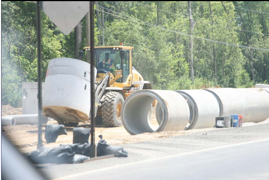
Crews installing new storm sewer along IL Route 62 as part of the LMP Section D – E/O IL 25 to IL 62 contract
