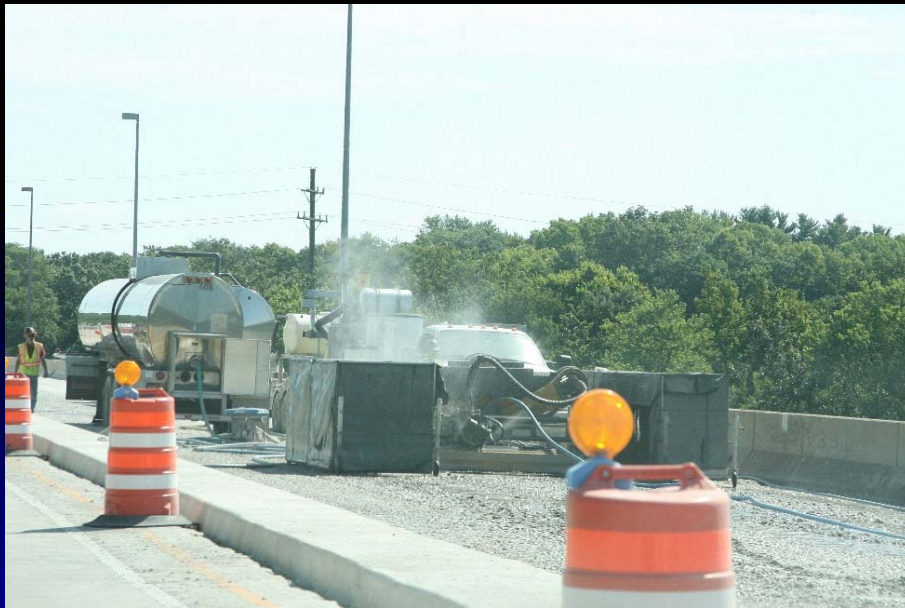
Crews removing the old worn out deck and repairs to parapet walls and substructure on the Fabyan over Fox River Bridge improvement project
