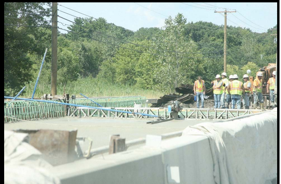
Crews place the rebar reinforcement mat and then complete the concrete pour for the new bridge deck on the Silver Glen over Otter Creek bridge replacement project
