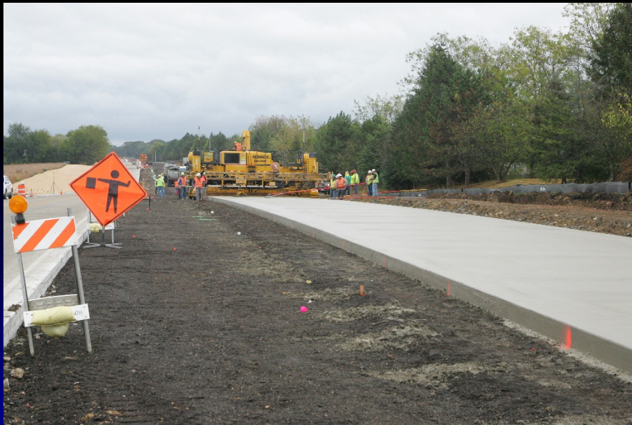
Semis and ready mix trucks feed the paving machine on the third concrete pour for Longmeadow Parkway
