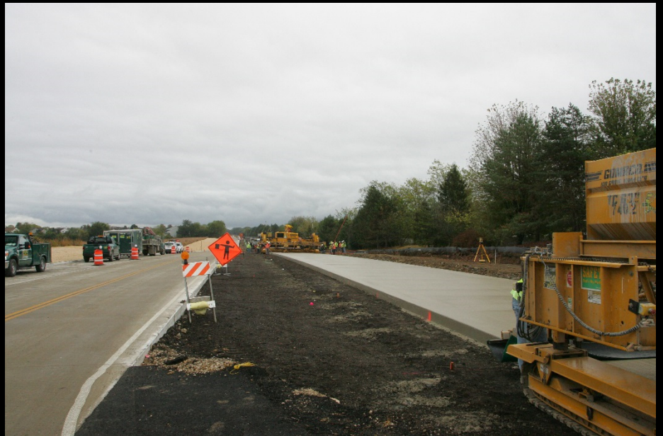
Semis and ready mix trucks feed the paving machine on the third concrete pour for Longmeadow Parkway
