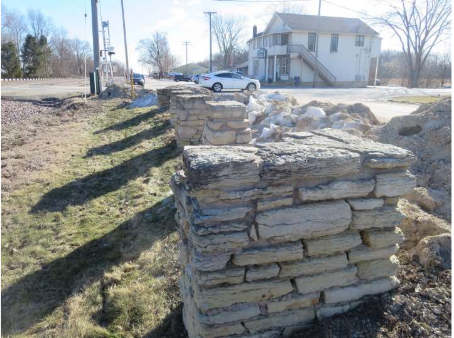
FIGURE 4: HISTORIC FOUNDATION PIERS AT THE ORIGINAL SITE.
