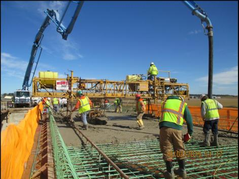
Crews placing the concrete deck on the new bridge over the UPRR tracks and the Metra Yard as part of the Anderson Road project.
