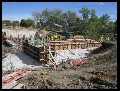
Crews demolishing the old bridge and preparing the new abutment as part of the Jericho Road over Blackberry Creek Bridge Replacement project
