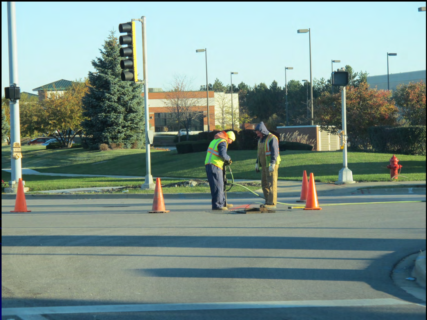
Workers modify electrical handholds for the Pace Route 529 Randall Road improvement project.
