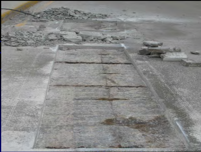
Workers complete deck patch repairs to the Kirk Road over UP RR bridge.
