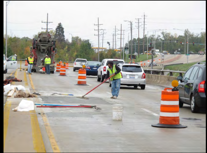
Workers complete deck patch repairs to the Kirk Road over UP RR bridge.
