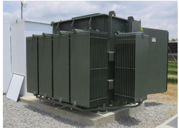
Figure 6. 3.2 MVA Inverter Step-up Transformer containing 575 gallons of oil
