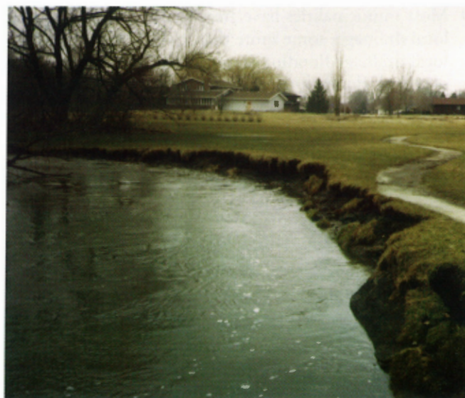
Streambanks in need of stabilization
