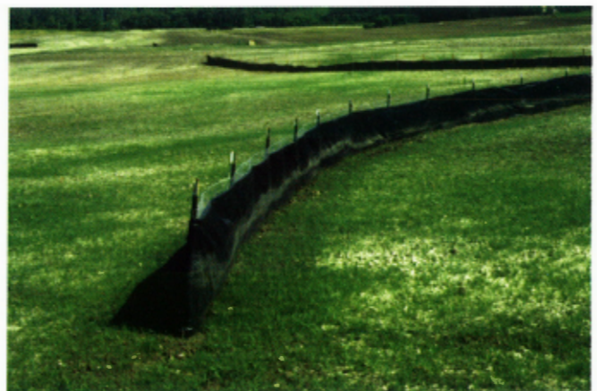
An example of silt fencing
