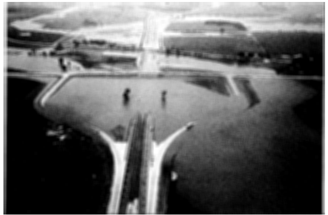
July 1996 flooding looking west along I-88 at Orchard Road in the Aurora area
