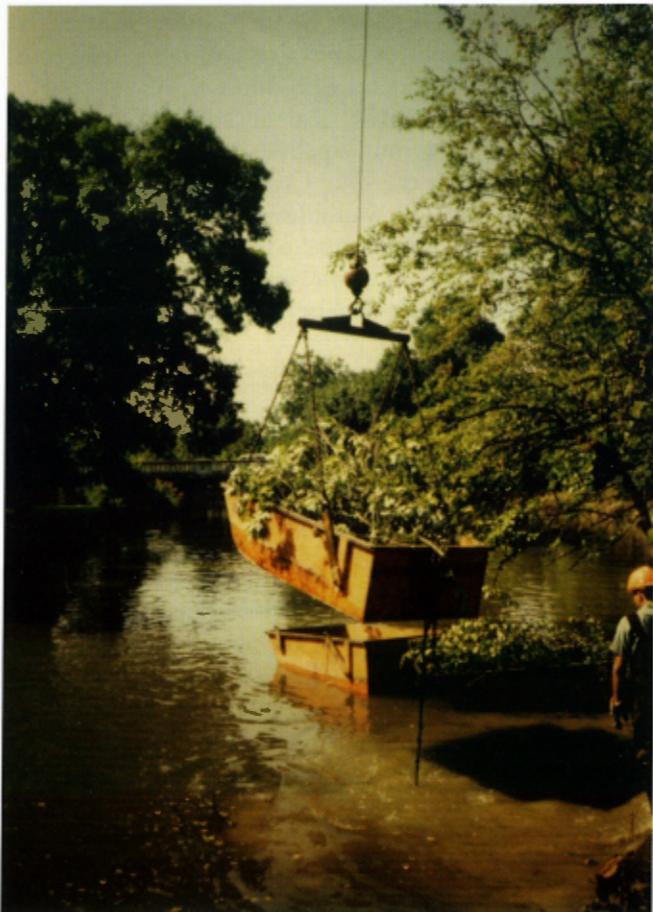
Removal of debris during stream maintenance demonstration project
